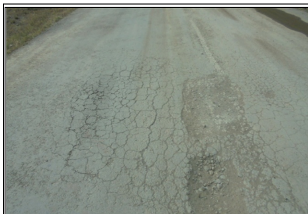
Fair Condition of Pavement
